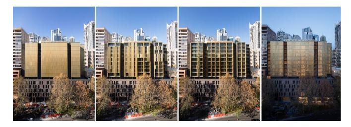
When the late afternoon sun hits the façade of Tzannes' newest mixed use residential and commercial building on the western perimeter of central Sydney, Australia, its more than 1150 anodized aluminium mesh shutters glow pure gold, softly filtering the light into the apartments behind and illuminating the precinct below. [See animation link below].
